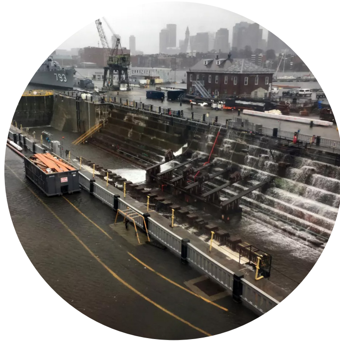
Naval Heritage and Critical Infrastructure at Risk: Flood waters pour into Dry Dock 1 during a record storm in 2018. Photo credit: National Park Service
